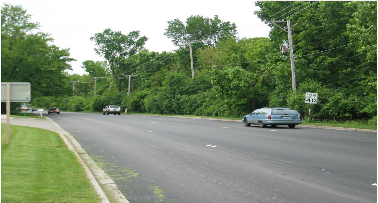
Northbound IL RTE 25; No existing pavement markings due to new resurfacing
