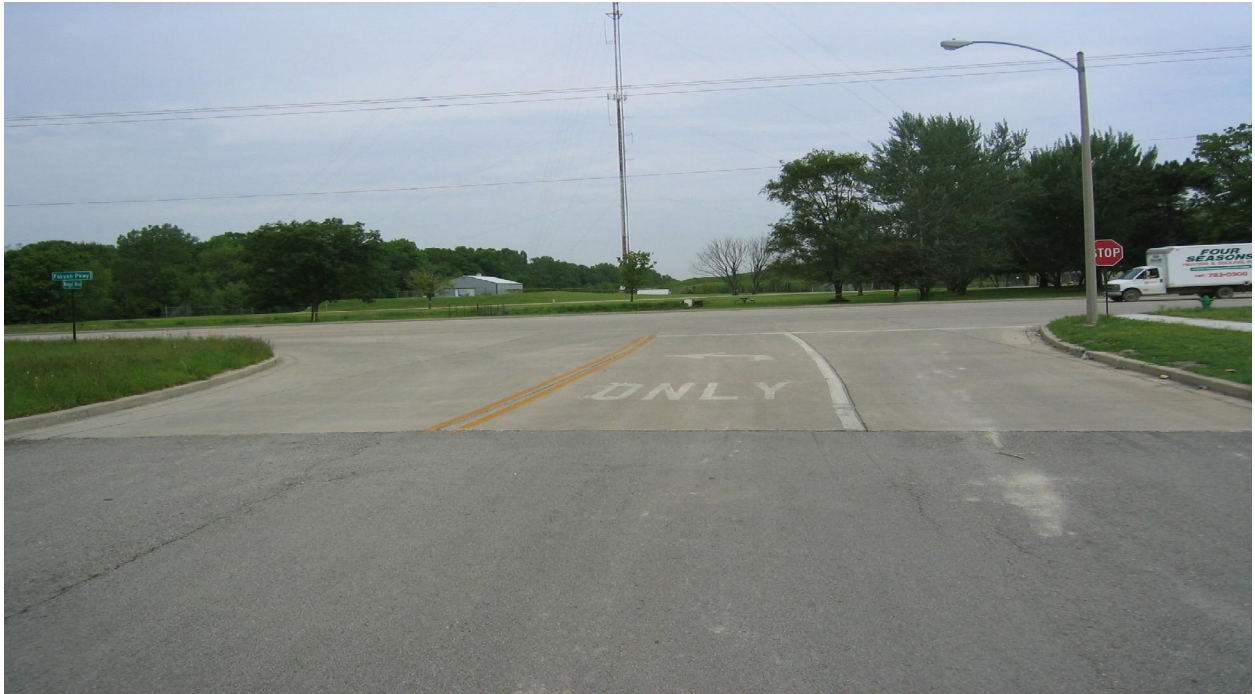
T-Intersection of Nagel Boulevard and Fabyan Parkway (Looking North)
