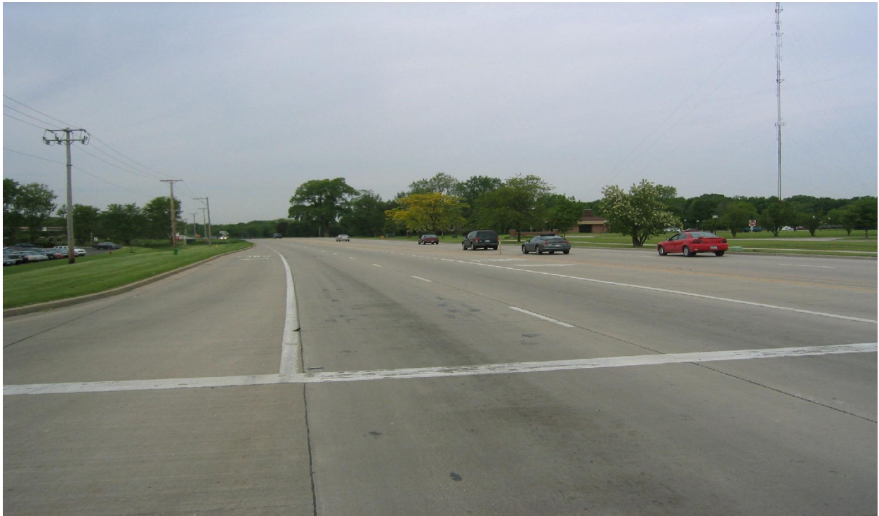
Eastbound Fabyan Parkway and Turn Lanes at North Raddant Road
