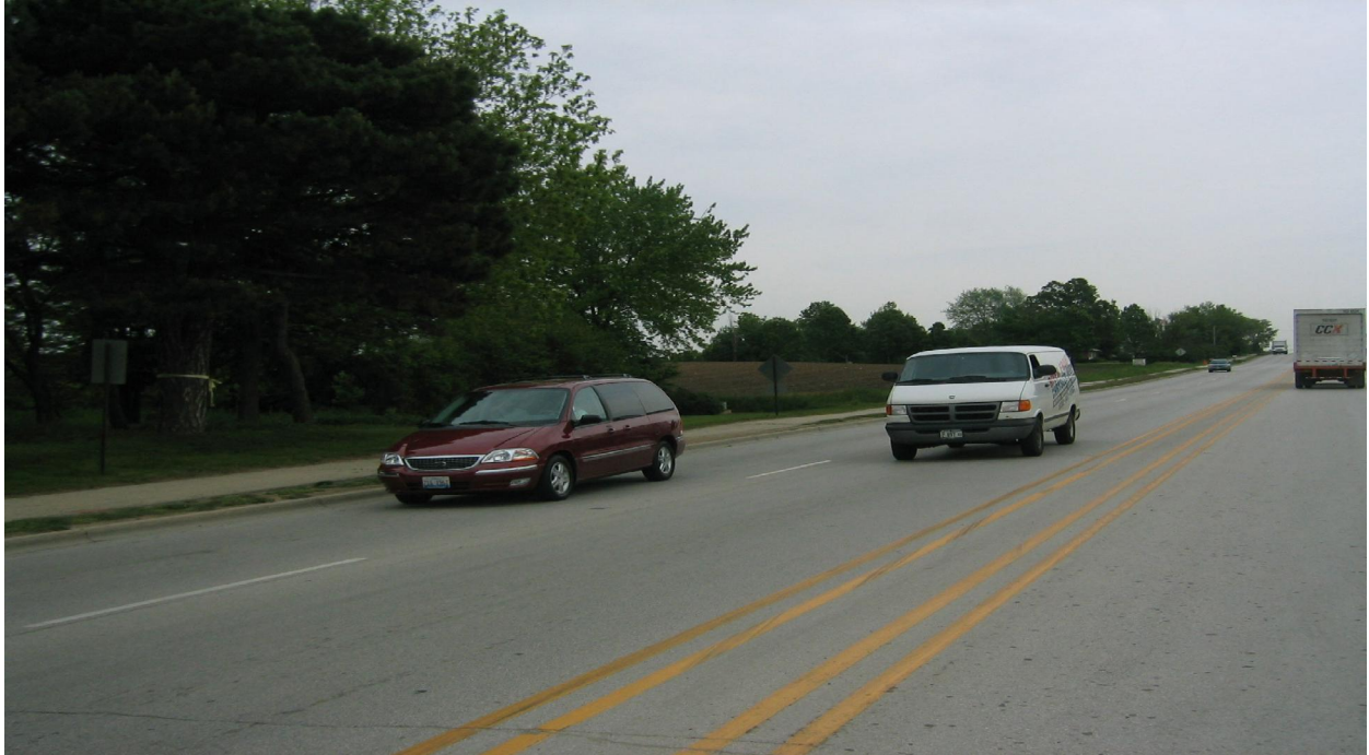
Westbound Fabyan Parkway at Kingsland Drive
