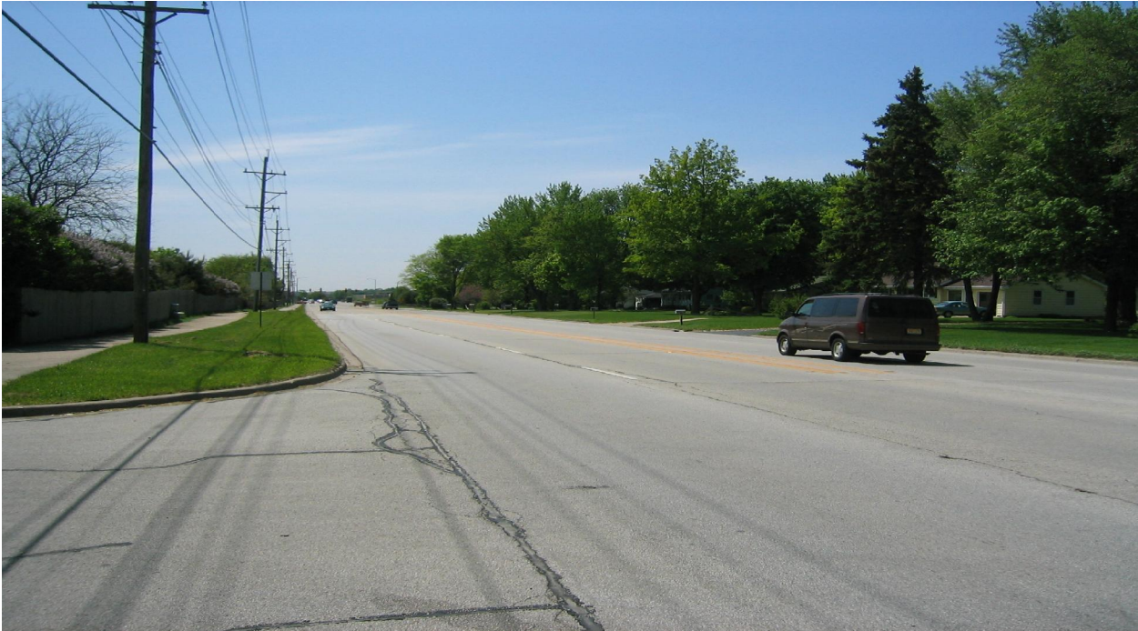
Eastbound Fabyan Parkway at Carriage Drive
