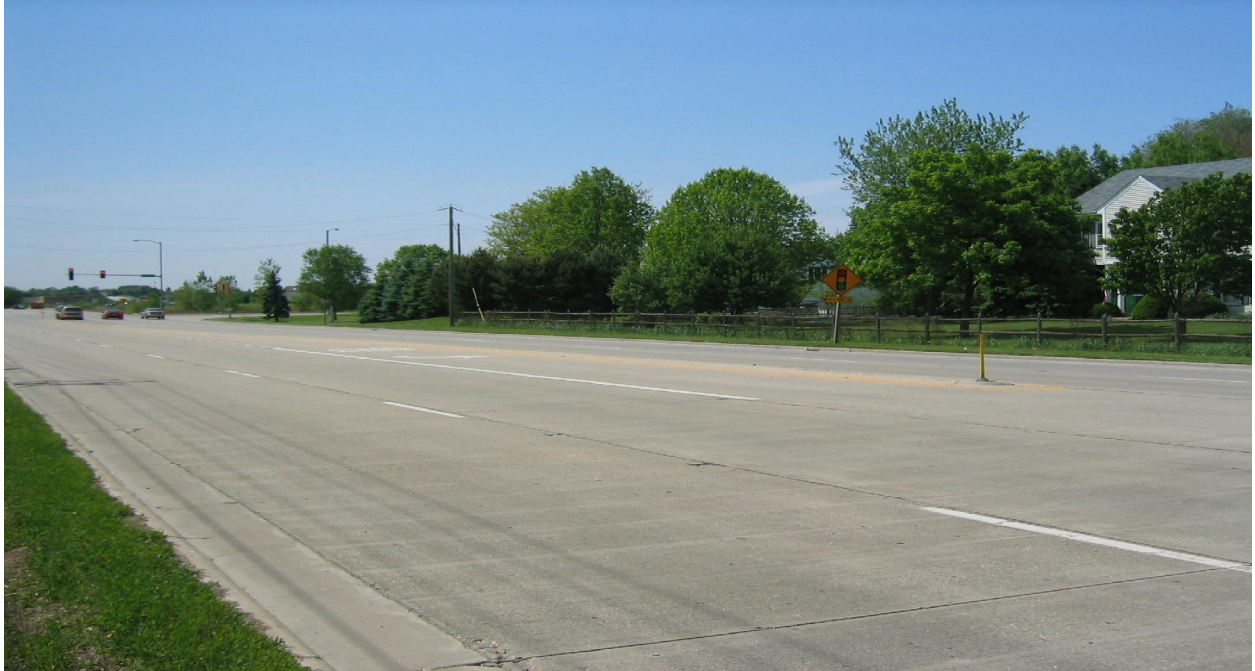
Eastbound Fabyan Parkway, Left Turn Lane and Raised Median at Heather Lane
