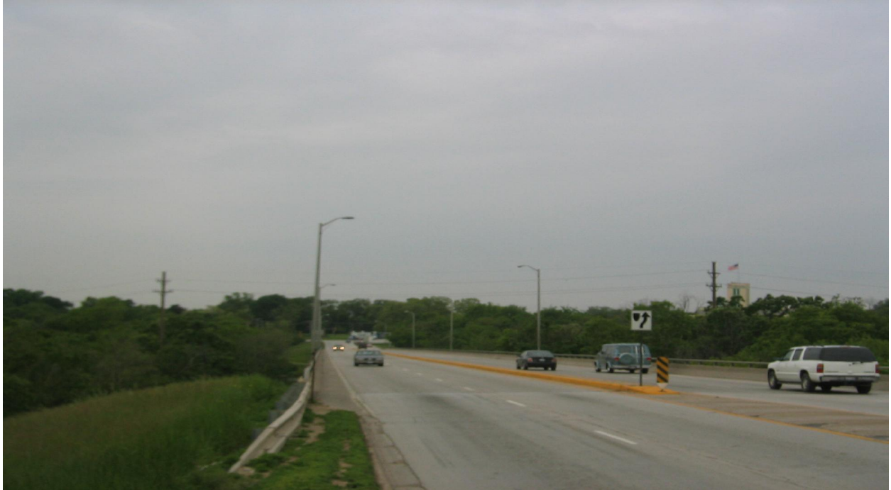
Facing Eastbound Traffic on the Fox River Bridge near IL RTE 25
