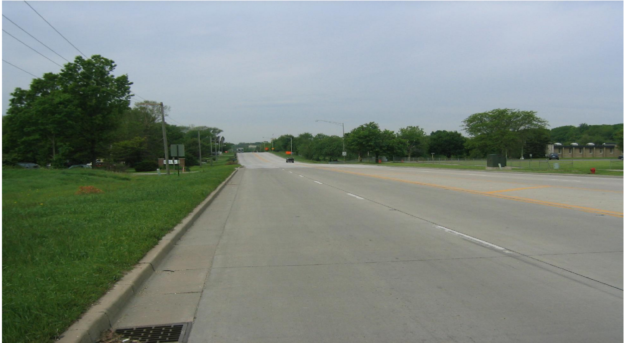
Eastbound Fabyan Parkway at Nagel Boulevard
