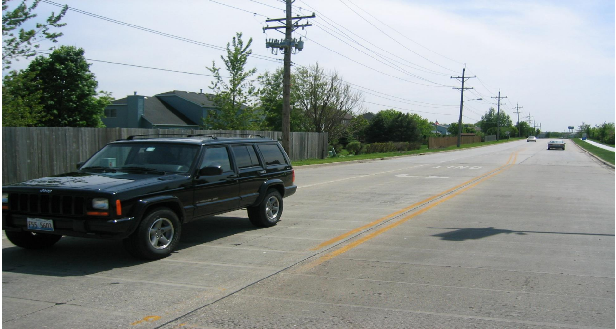
Northbound Western Avenue South of Fabyan Parkway
