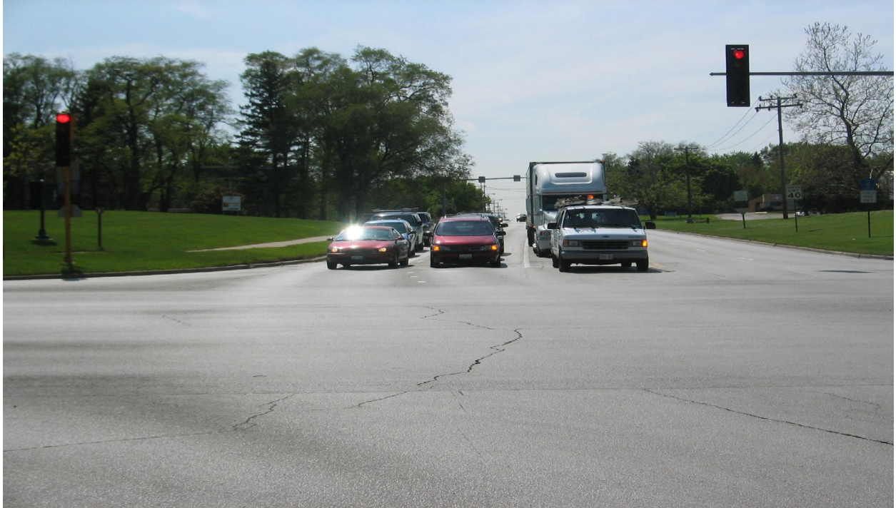
Eastbound Fayban Parkway at IL RTE 31 (Batavia Avenue)
