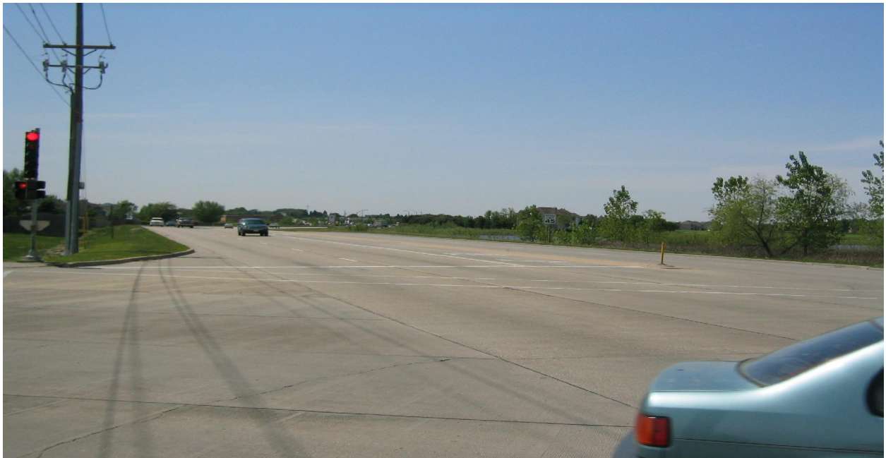
Eastbound Fabyan Parkway, Left Turn Lane, and Raised Median at Western Avenue.
