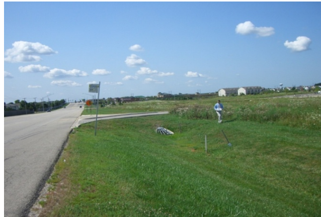
Route 529 bus stop without landing and walkway
