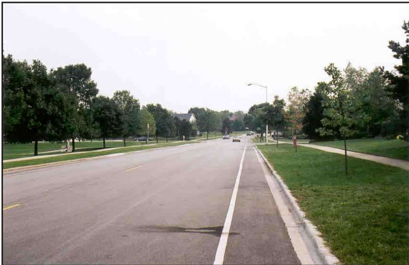
Closed Drainage - Bike Path
