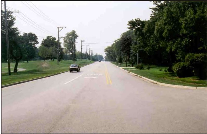
Three-Lane Cross Section
