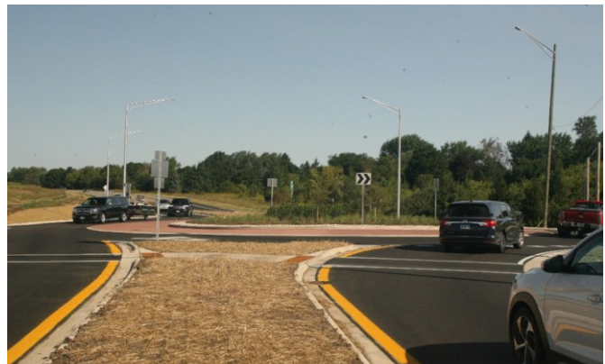
Burlington Road at Bolcum Road Roundabout
