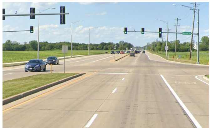
Orchard Road Corridor Improvements
