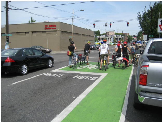
Bike boxes allow cyclists to move in front of the travel lane in order to be more visible to cars and avoid turning conflicts. Politicians in Portland, OR are advocating an increase in bike box construction as a safety measure in the wake of cyclists fatalities at intersections.
